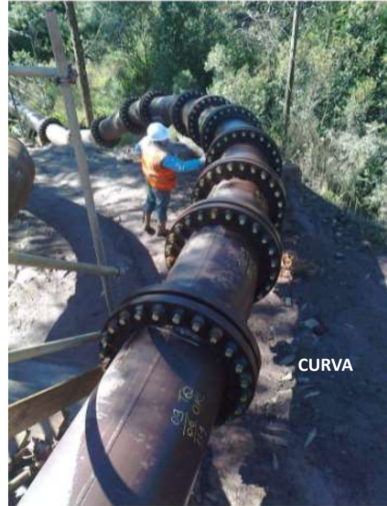
Figure 4. Unorthodox changes in direction in a large diameter flanged lined tailings pipeline
